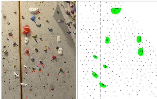
**Figure 11.** (Left) White holds forming our replicated route were positioned by finding optimal matching against T-nuts permanently installed in the gym wall. (Right) T-nut positions are shown as blue circles. Red circles correspond to hold centers and crosses correspond to the optimal T-nut match.
