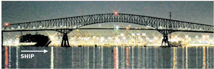
1:27 A.M. The ship changed direction as it neared one of the bridge's piers.
