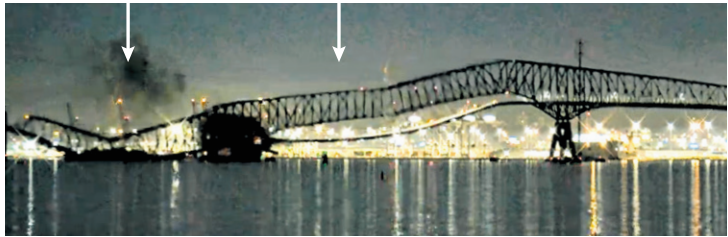
1:28 A.M. The northern span began to collapse seconds later.
