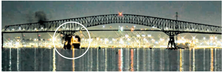
1:28 A.M. Southern and central spans collapsed within seconds of impact.
