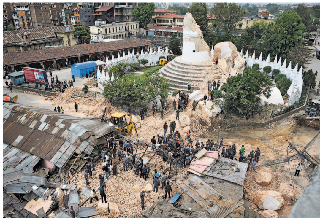
Many people died when the nine-story Dharahara Tower, a tourist spot in Katmandu, collapsed.
